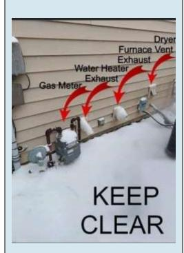
When you're out clearing your driveway, take a moment to look at these to make sure they are clear from snow and ice. Blocked exhaust vents or redirecting exhaust fumes to furnace intakes is a common cause for Carbon monoxide in a household.
